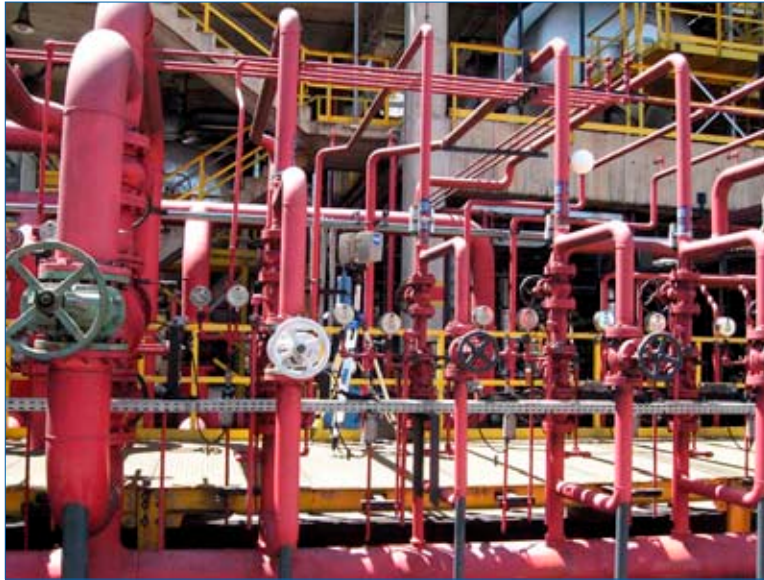
3D Laser Scanning in chemical facility
